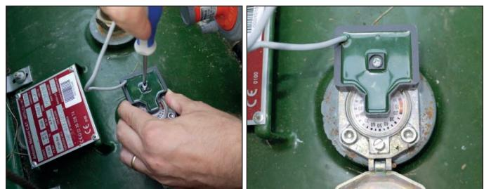
Using potentiometric/ratiometric sensor, replace the gauge pre-existing with the new probe.
